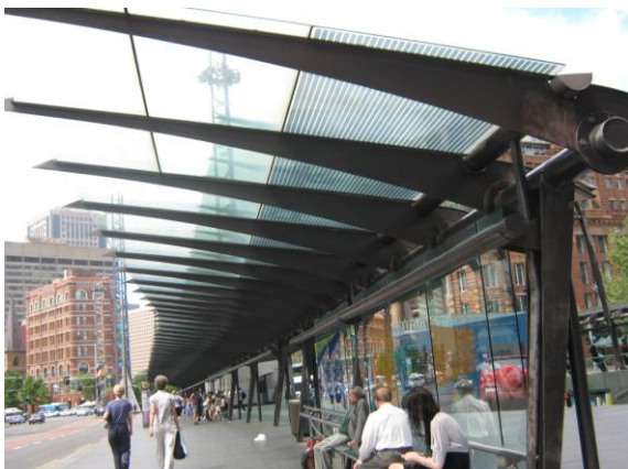
Figure 12: Bus stop with Cantilever Roof.
