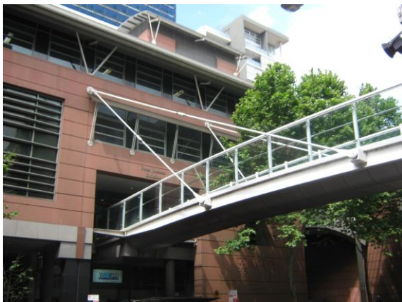
Figure 10: Pedestrian bridge joining two UTS buildings: member in tension and bending.
