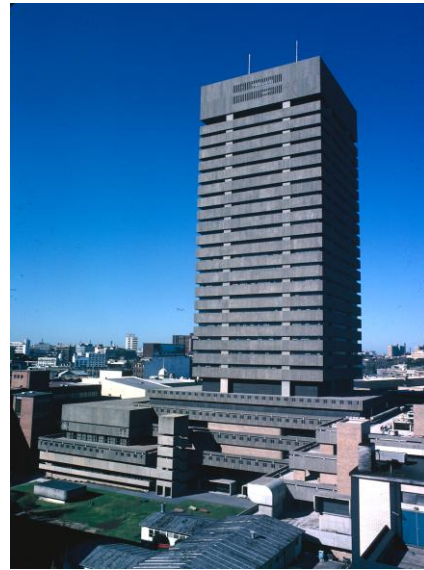
Figure 9: UTS Tower (R.C. Framed Structure).
