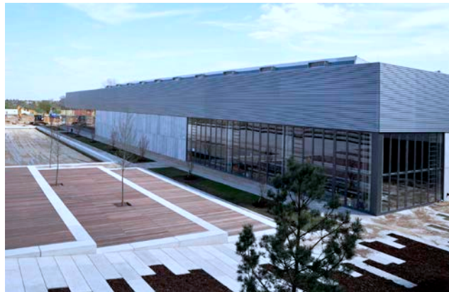
Figure 1: Solarlux Campus in Melle - production hall 3.
