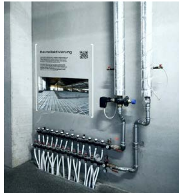
Figure 3: Display with a photo documentation taken in the construction phase.
