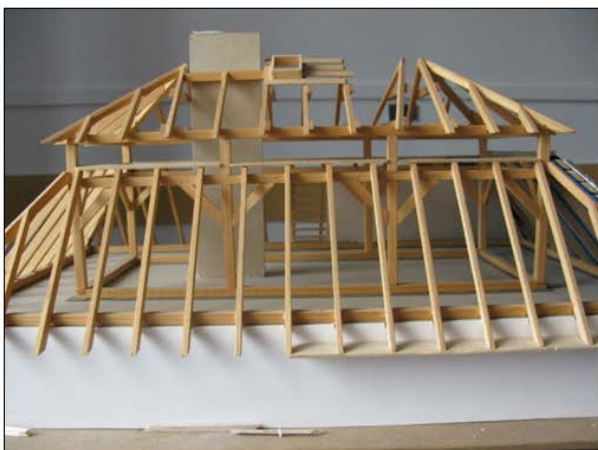
Figure 5: The pictures show preliminary models of Cracow mansard roof made by first-year students at the Faculty of Architecture, CUT, in the design classes of General Building Engineering.
