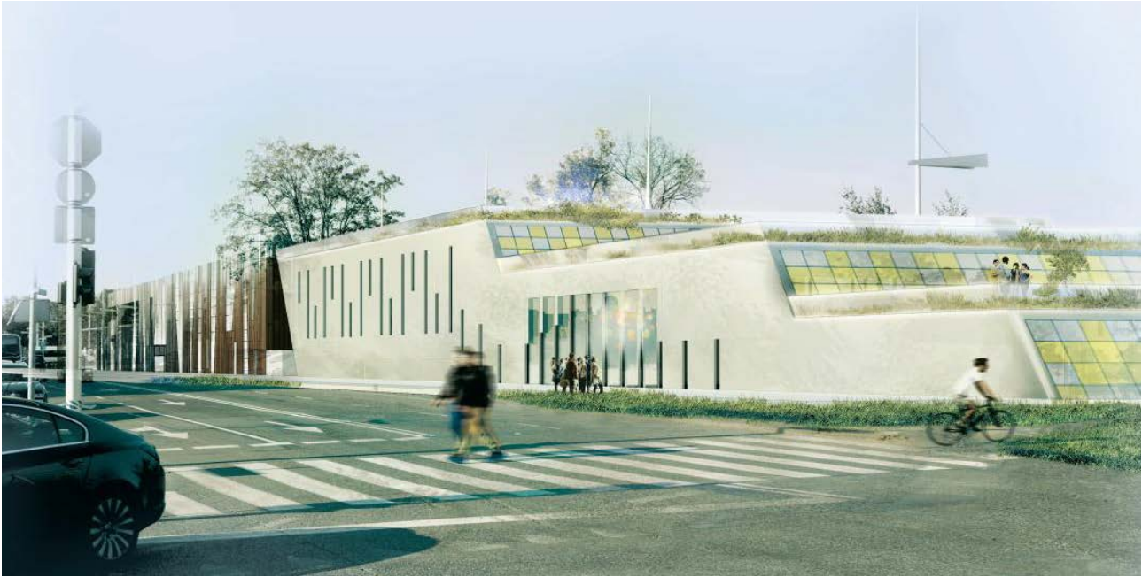
Figure 2: The main façade of the existing Copernicus Science Centre and the newly designed building (students: A. Koziol and M. Tomaszewska, Master's studies, Semester 1, 2014/2015, the Faculty of Architecture, WUT).
