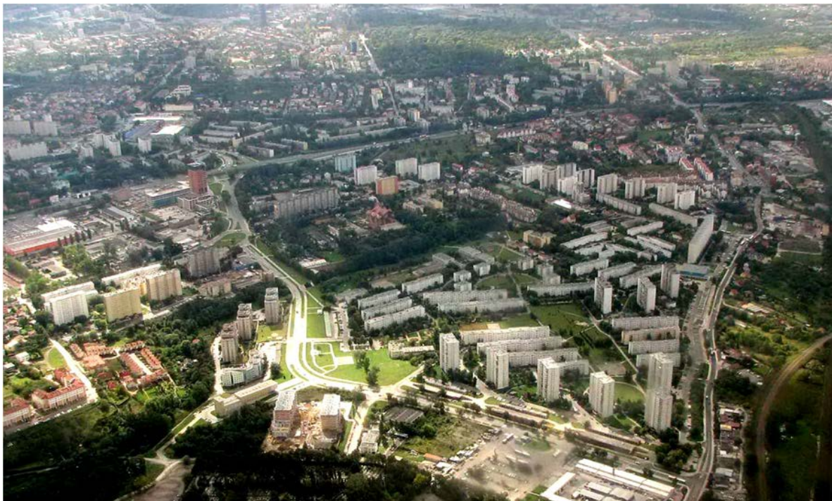
Figure 1: Flat roofs are a typical element of the landscape of contemporary cities. (Kraków, Poland - photo by R. Marcinkowski, 2007).
