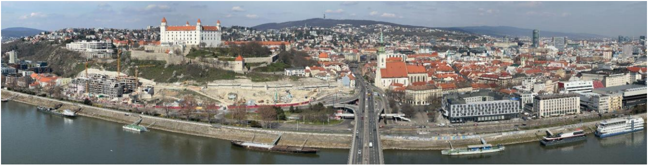
Figure 3: Panoramic view of the Castle Hill in Bratislava, Slovakia. On the left, next to the bridge exit under the castle, a large part of the hill mass for the Vydrica development project has been dug away. According to the ecological algorithm, the excavated material should be used in the construction. The enormous volume of excavation for this project required a large amount of energy to remove the hill-mass created by nature (Photograph: R. Špaček).
