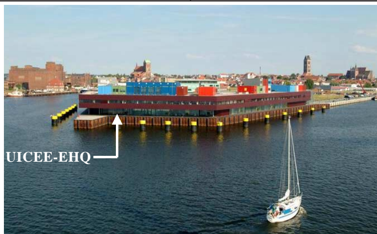
The modern TGZ building, which houses the UICEE-EHQ office.
